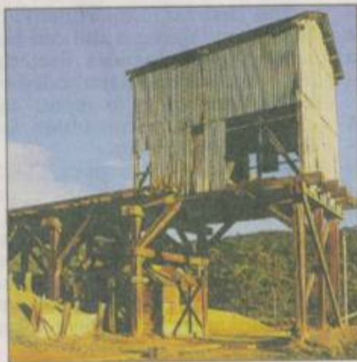
"SAFETY RISK" : The restored railway ore loader was demolished on Monday.
